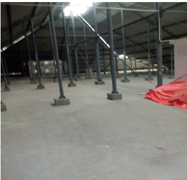
Figure 5 - The attic space
